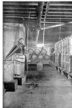
Part of the Cold Storage Room, Showing the Large 100 Gallon Perfume Tanks
