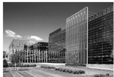
Global Research & Development Center, Suffern, NY.
